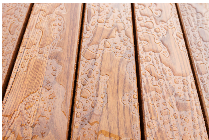
Final coat on wood panels
